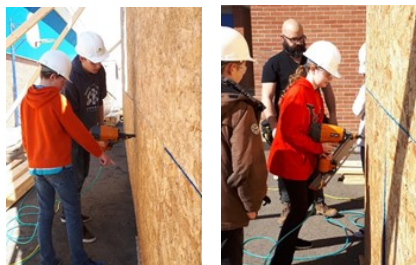
Working on our "Tiny House"
